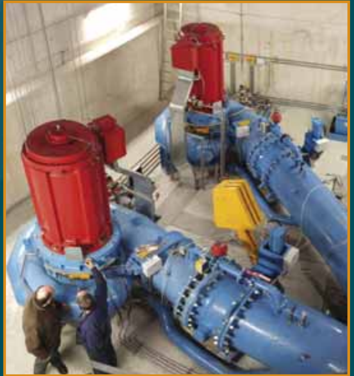
Hydropower plant with two twin parallel generators in operation
